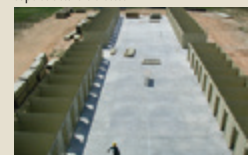
After the superstructure is erected but before the building is enclosed
